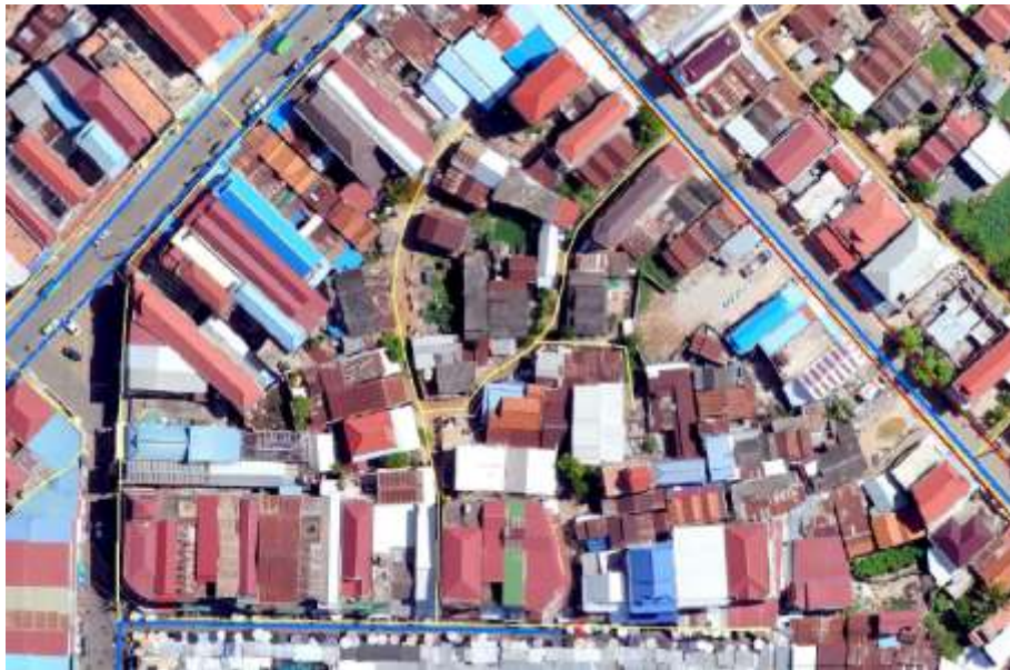
Figure 3 Collector line installation in very high density area
