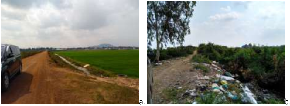
Figure 13 Raised road at site of WWTP access road
