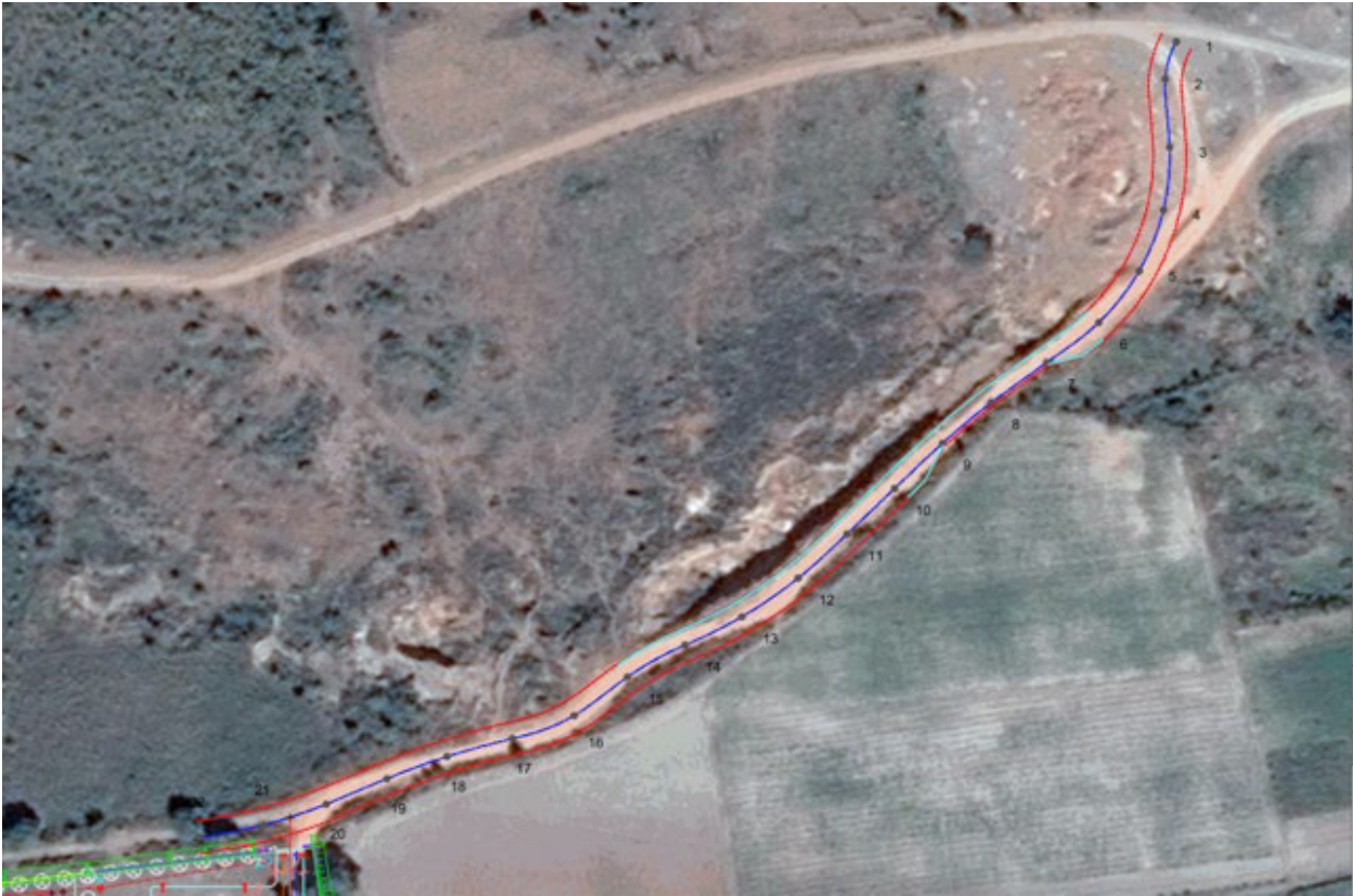
Figure 6 Overview of Landfill Access Road (source: PMC)
