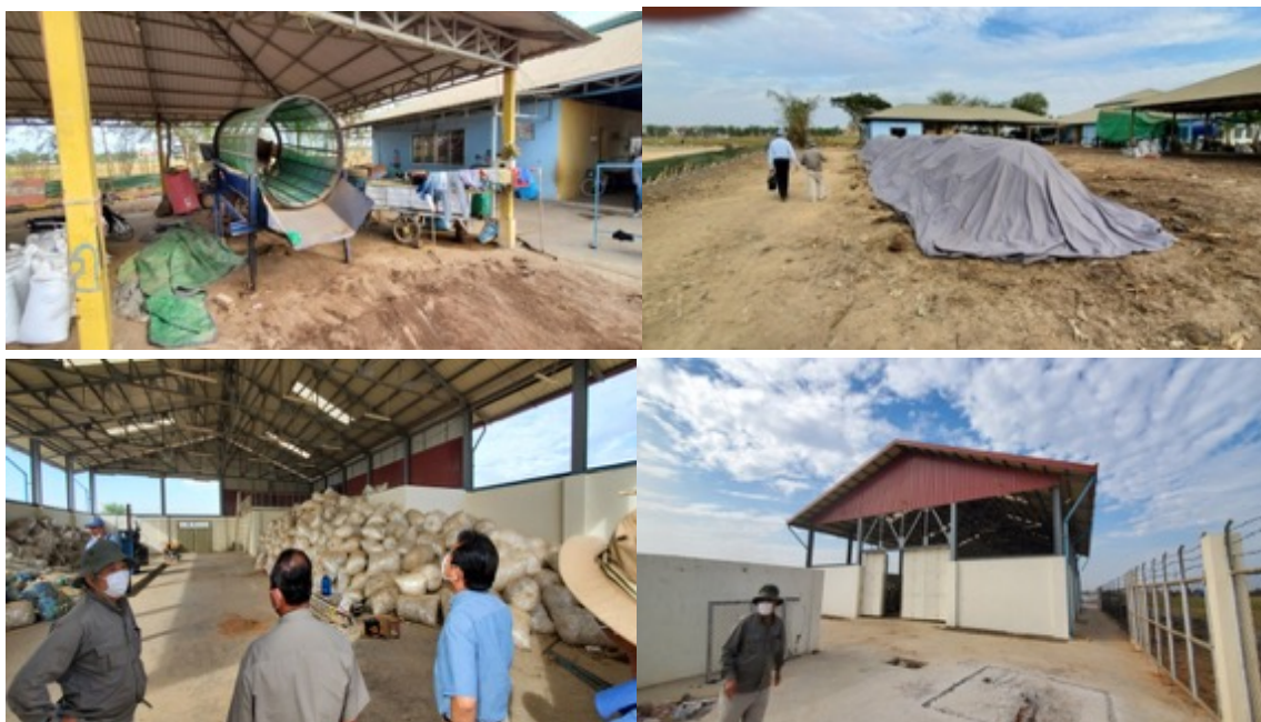
Picture 2 Composting Plant at Existing Dumpsite (source: PMC)
