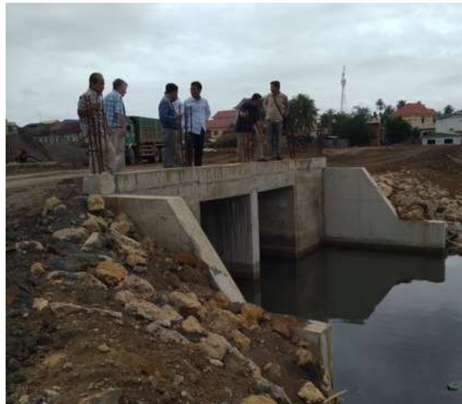
Drainage Outlets Locations No. 1
