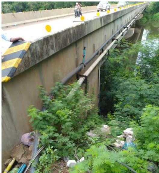
Drainage Outlets Locations No. 2
