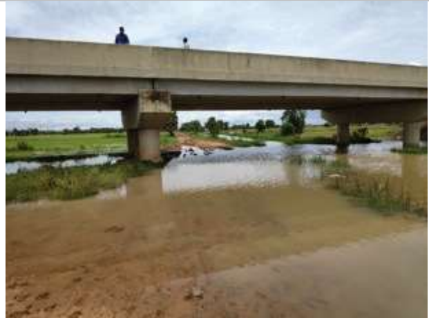
WWTP access road under a low bridge
