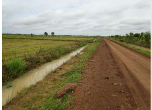
Access road to WWTP
