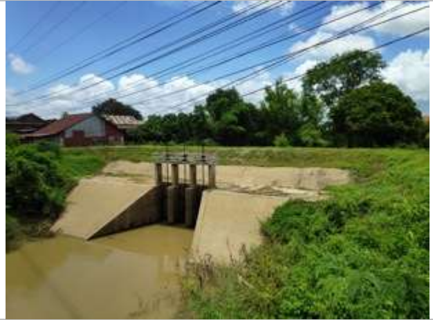
Existing sluice gate
