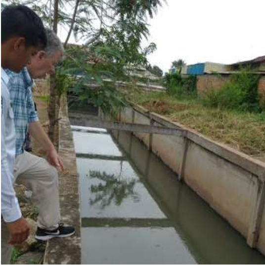
Existing Drainage Channel-Connected to above Outlet and Channel Extension
