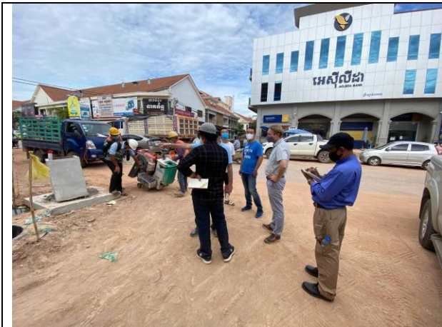
Site visit with Contractor, ongoing works under the "38 roads infrastructure development and rehabilitation"
