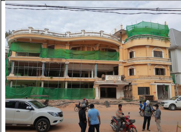
Hotel on project road under demolition to convert to supermarket
