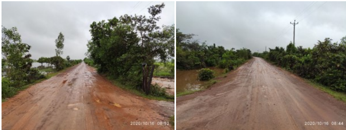
Picture 4 Access Road Key Sections in Middle and End of Road (source: PMC)
