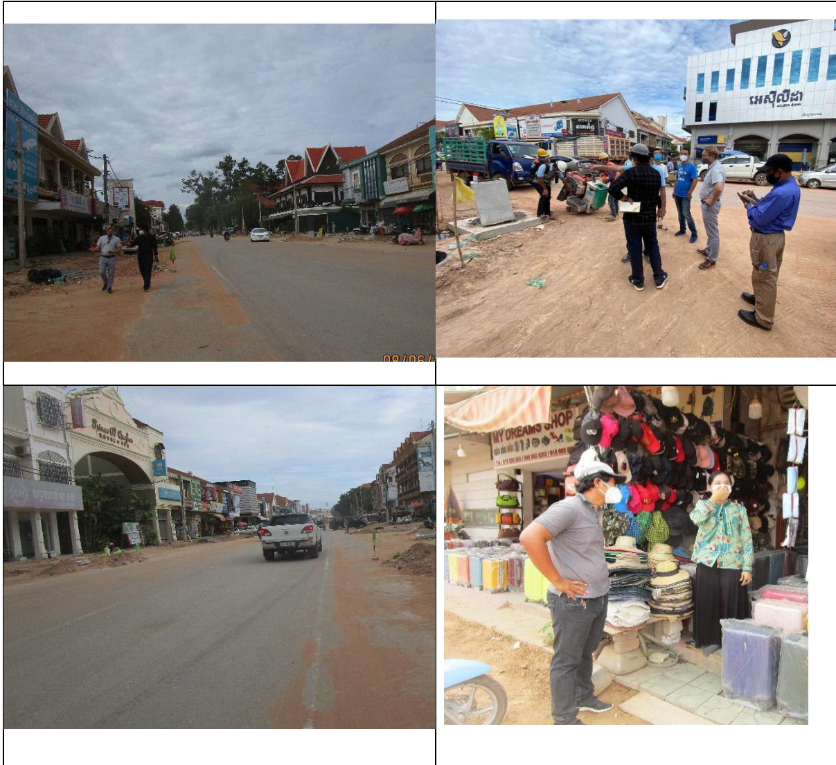
Siem Reap: Sivutha Boulevard conditions (June 2021) – the planned road works under the variation are dependent on the completion of the sewer and drainage connections under the 38 roads project
