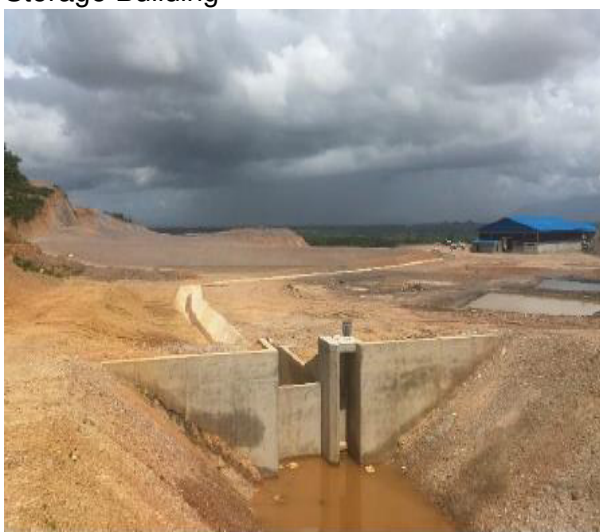
Water Intake Wier
