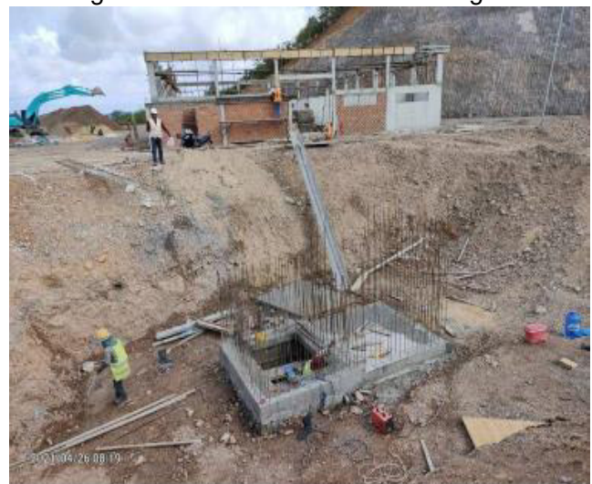
Construction of Septic Tanks near SRM Building
