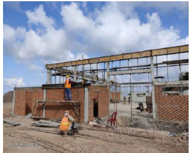
Building Roof Structure of SRM Building
