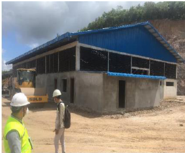
MRF Building 80% completed
