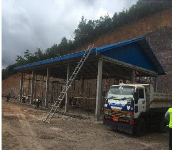
Structure and Roof completed – Roof Storage Building
