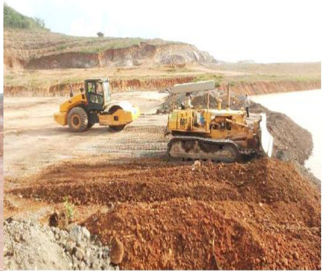
Photograph 3: Backfilling in Cell 2 of SWM Improvements
