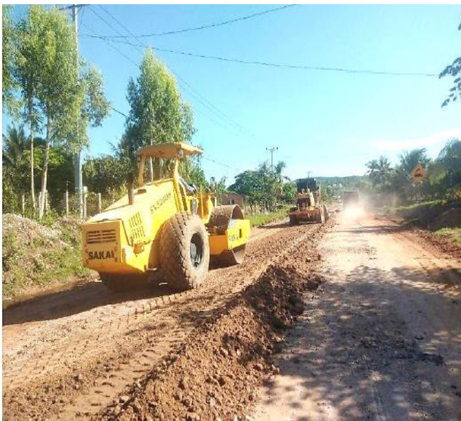
Photograph 4: Access road works in SWM Improvements
