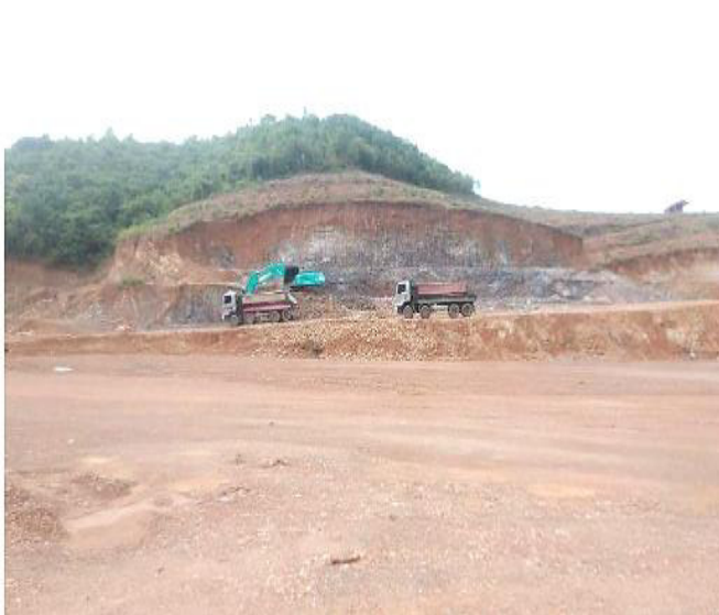
Photograph 2: Earthworks on Cell 1 of SWM Improvements
