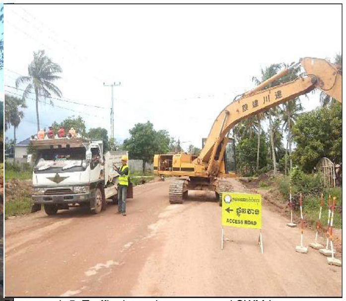
Photograph 5: Traffic detour in access road SWM Improvements
