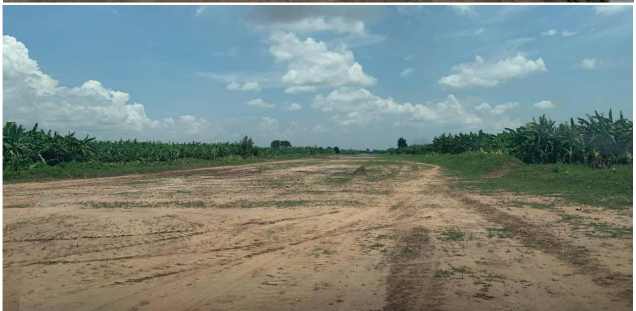
Picture 8 to 10: Improvement Road of Flood protect Neak Loeung subproject
