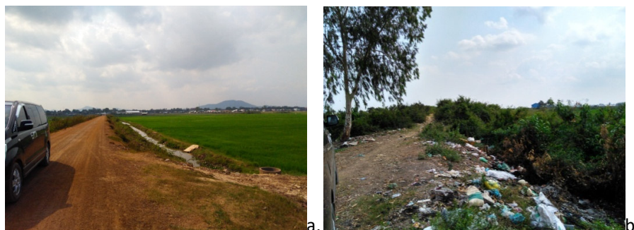
Figure 8 Raised road at site of WWTP access road
