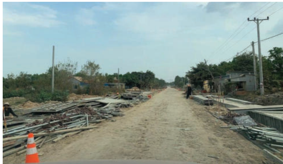
Picture 1 to 3: Road development of Bavet subproject
