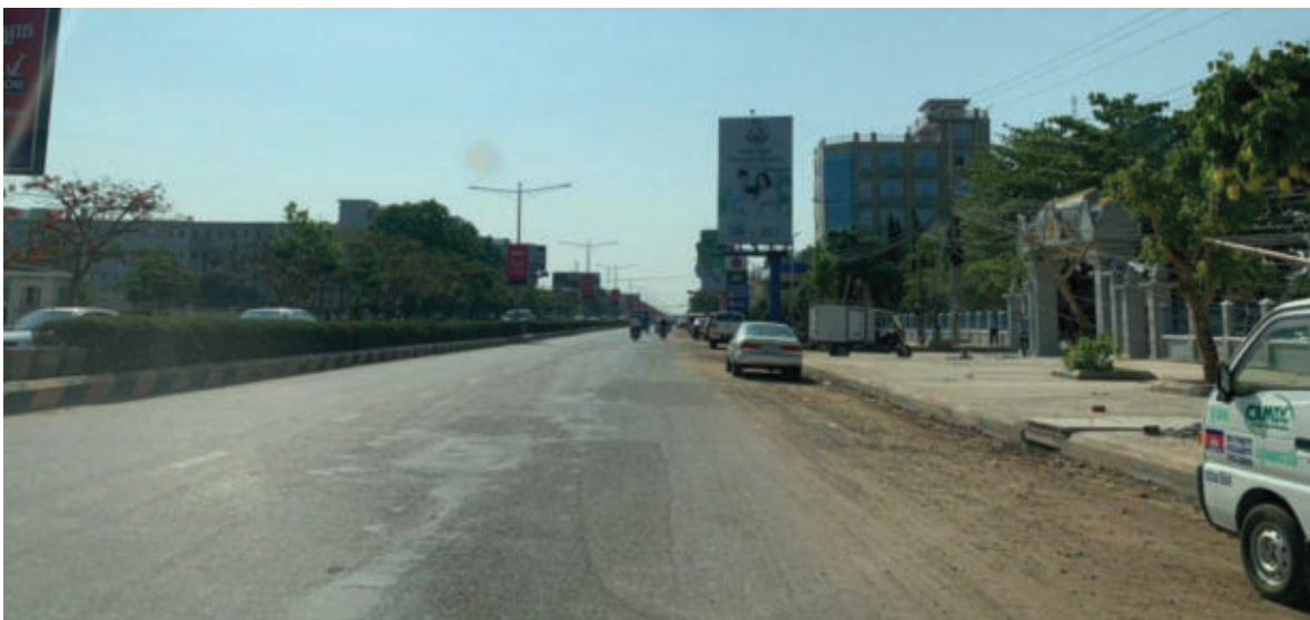
Picture 4 to 6: Wastewater Treatment system (Storm Damage) for Subproject in Battambang
