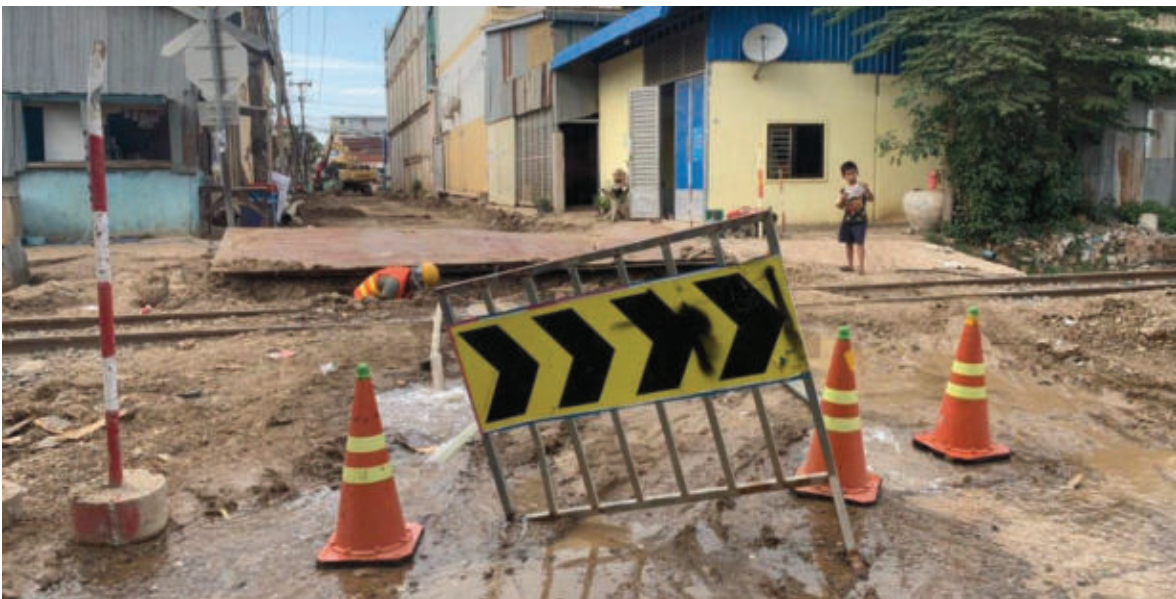
Picture 7 to 9: Poi Pet Subproject: Wastewater Treatment Subproject “Storm Drainage” (The Road and Drainage system are under construction)
