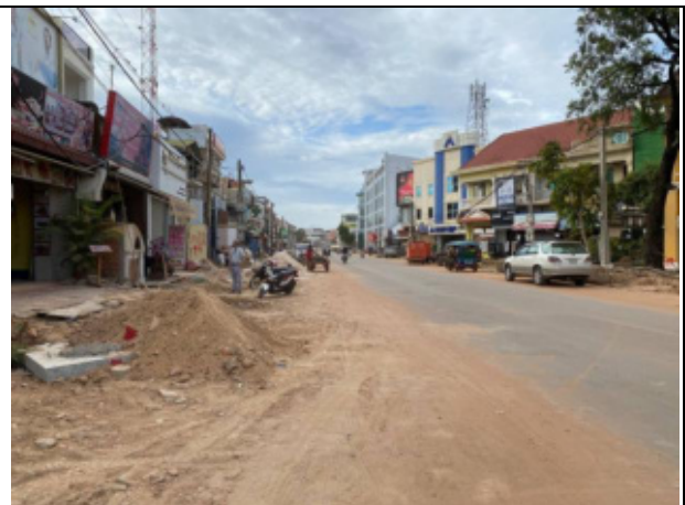
Ongoing works under the "38 roads infrastructure development and rehabilitation"
