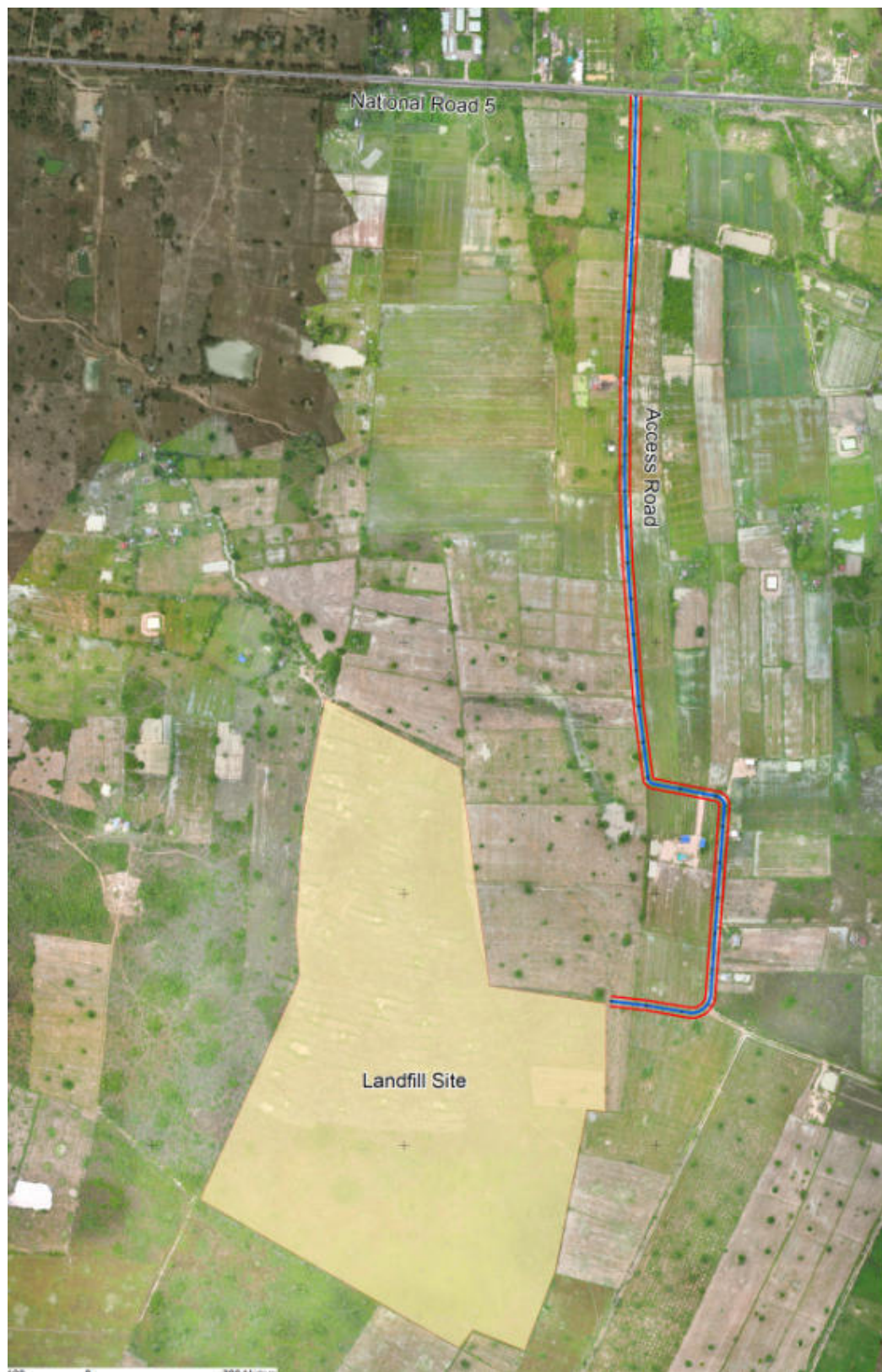
Figure 2 Pursat Landfill and access road
