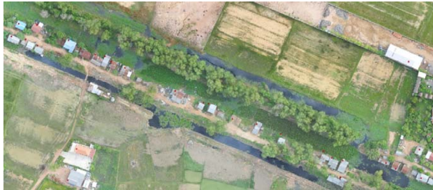
Pool of raw sewage between two existing outfall point of the drainage system in the defunct irrigation canal which formed at the start of the rainy season as backed up sewage is flushed out from the drainage network
