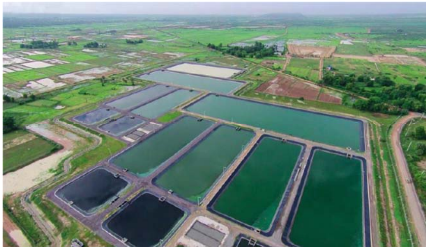
Figure 3: The Wastewater Treatment Station in Siem Reap
