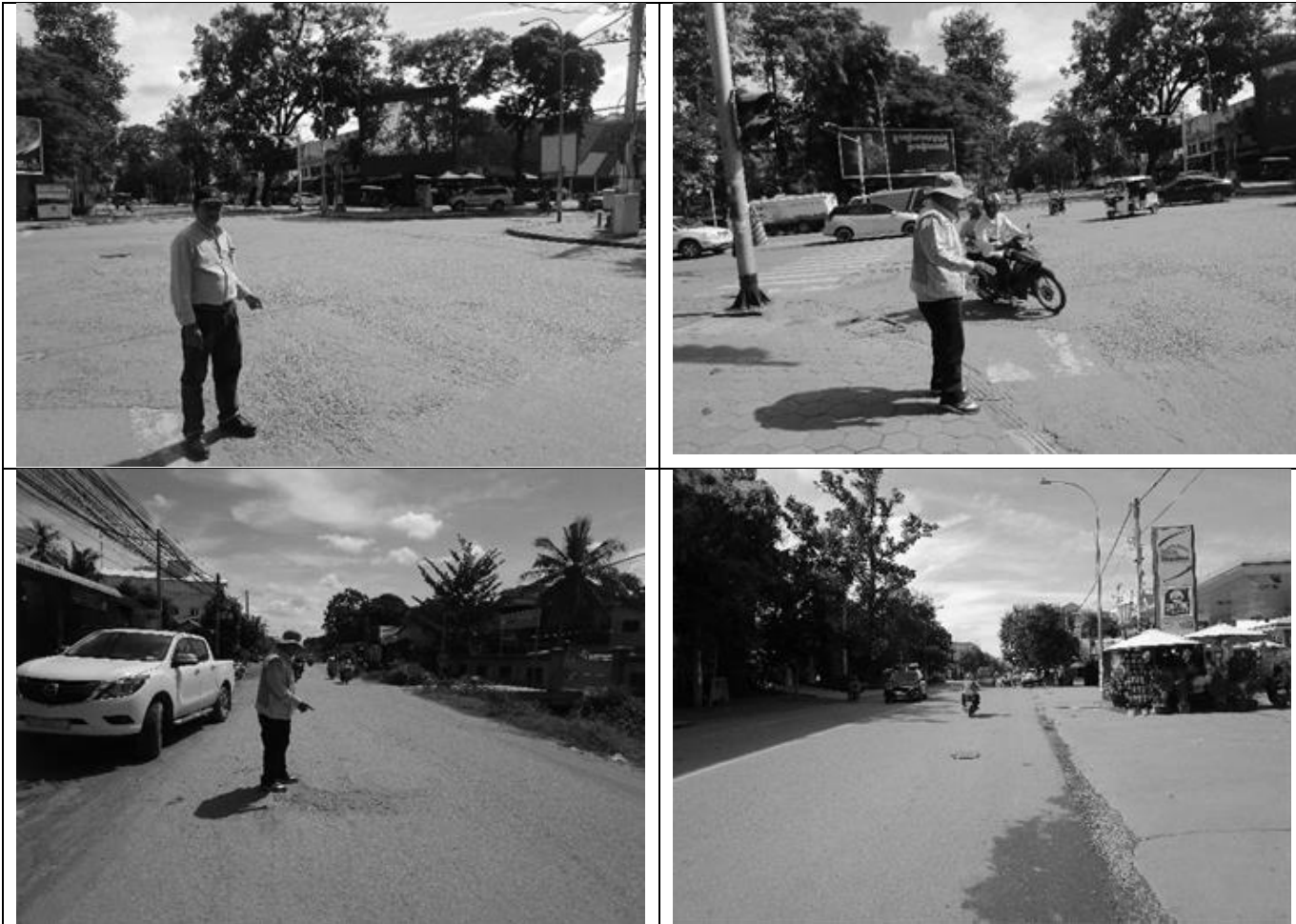
Siem Reap: The manhole sites in the roadway are well filled and maintained (September 2020)
