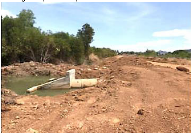
Coastal Road to be upgraded
