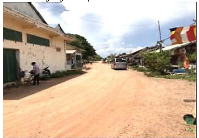
Part of Coastal Road improvement
