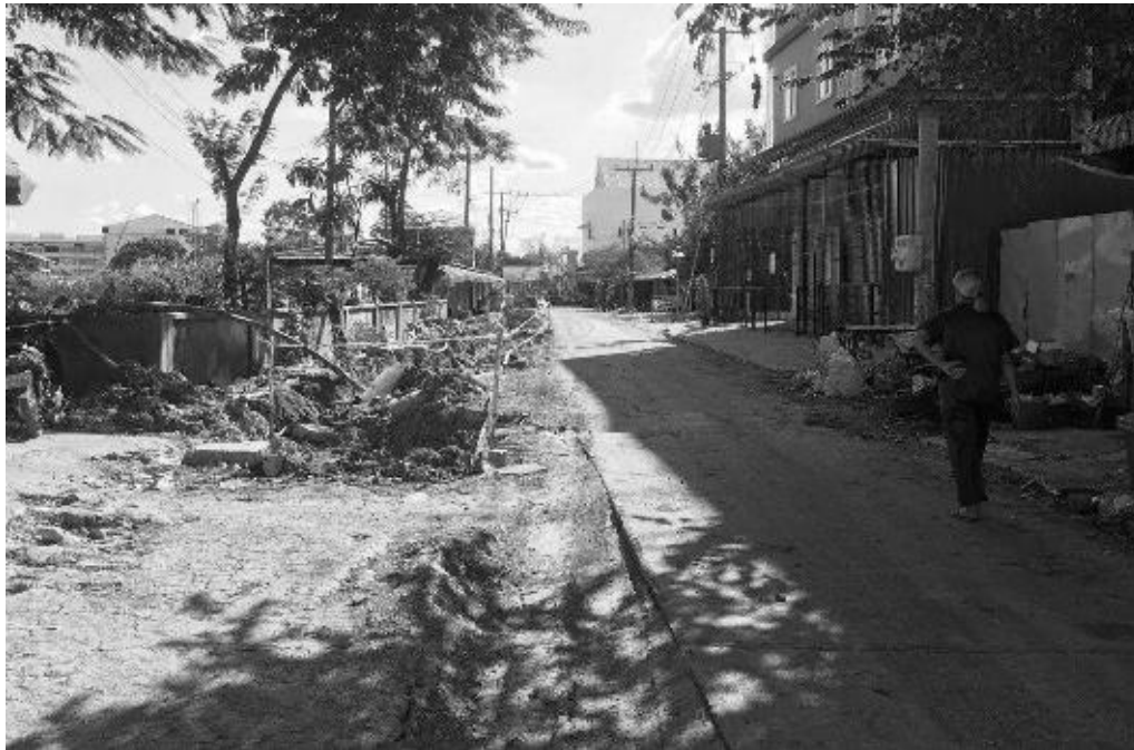
Picture 5, 6 &7: Poi Pet Subproject: Wastewater Treatment Subproject “Storm Drainage” (The Road and Drainage system are under the construction)
