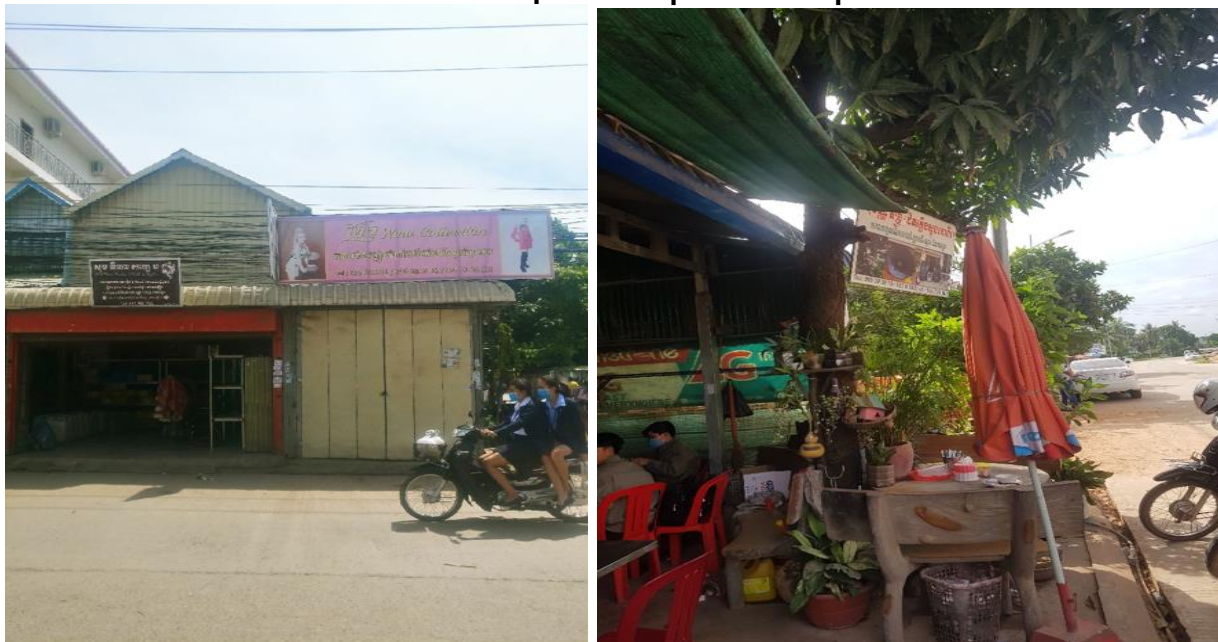
Picture 3.1: Examples of Impact on shop fronts
