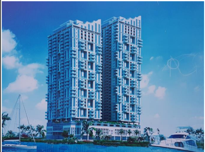
associated house/building connection complications
