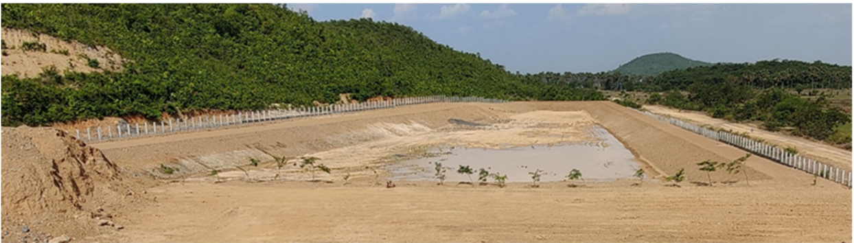
Completed rain water runoff balancing pond
