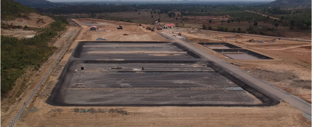
Overview completed asphalt lining of waste cells and leachate ponds
