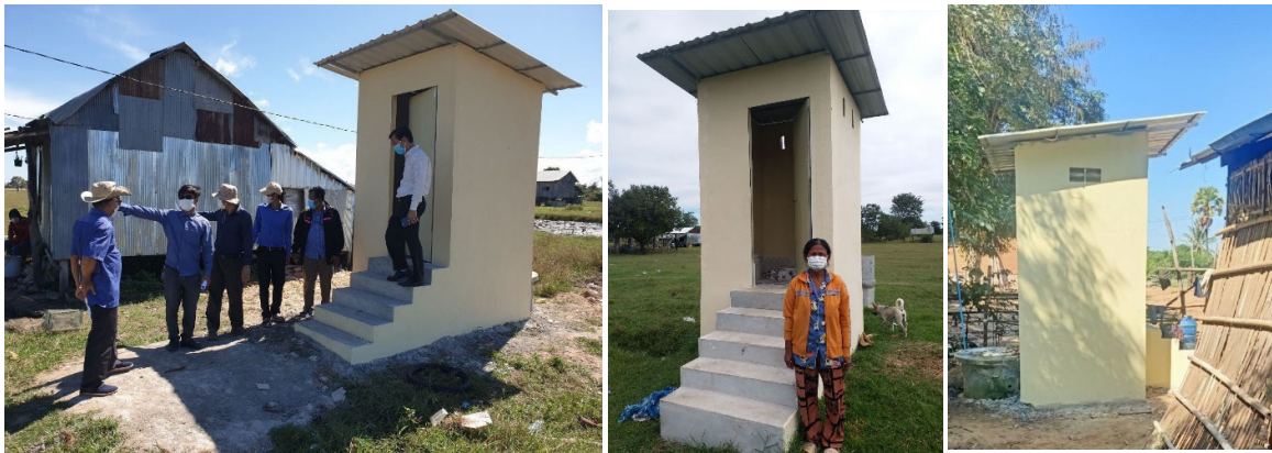
Completed VIP latrines
