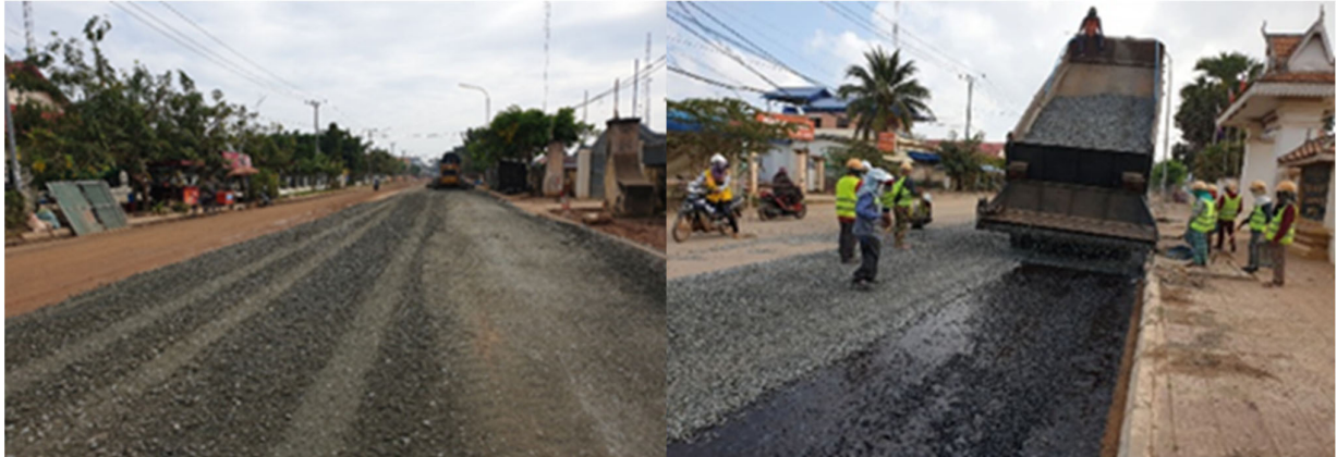
Pavement reinstatement; installation of a new base course and DBST layer
