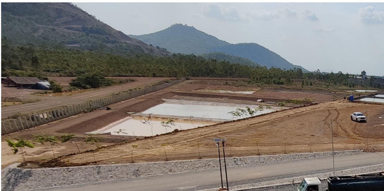
Completed constructed of wetland
