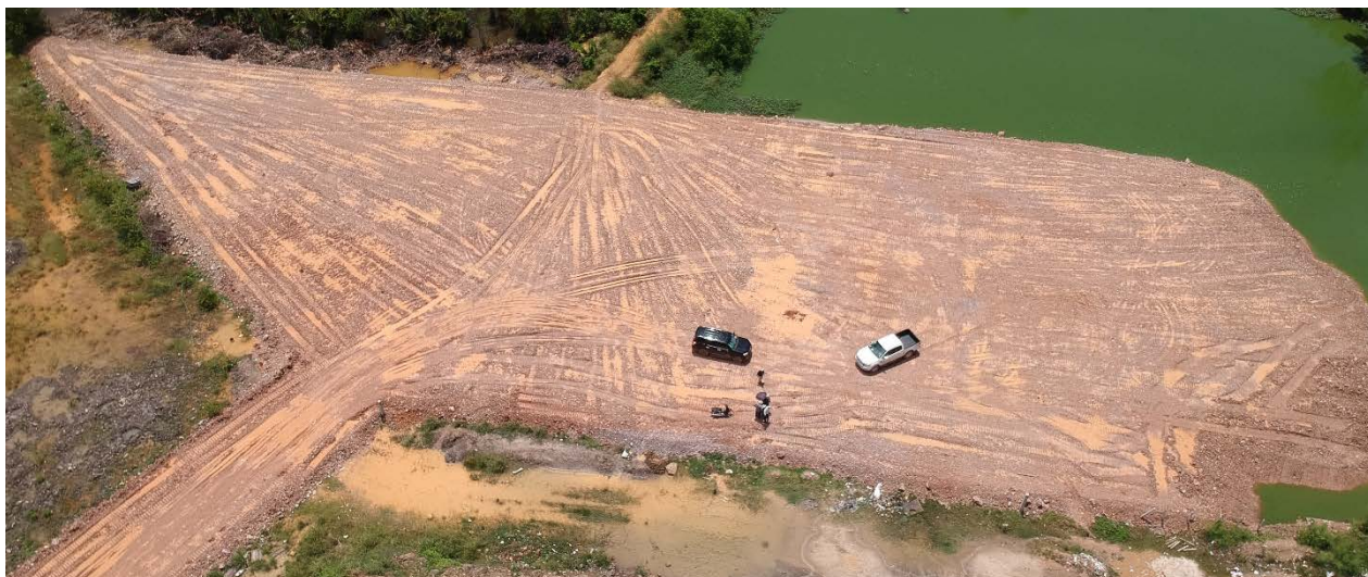
Soil filling of the MPS site and access road
