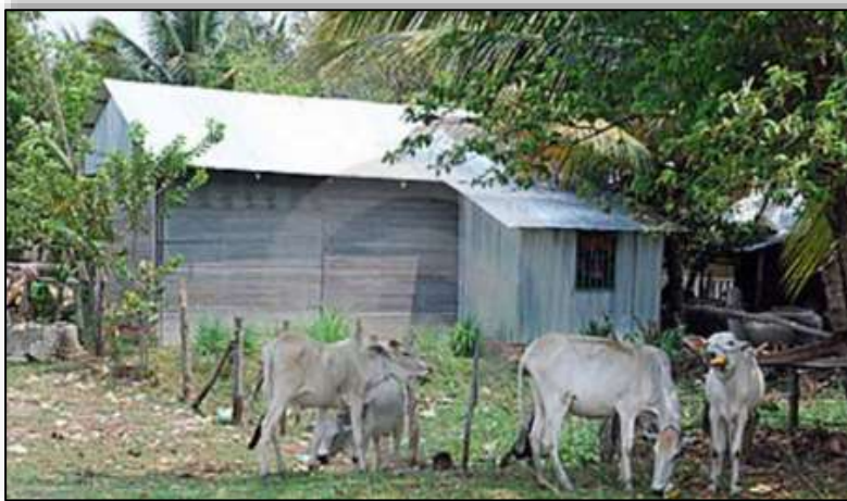
Figure 25-3 Metal sheet house on ground
