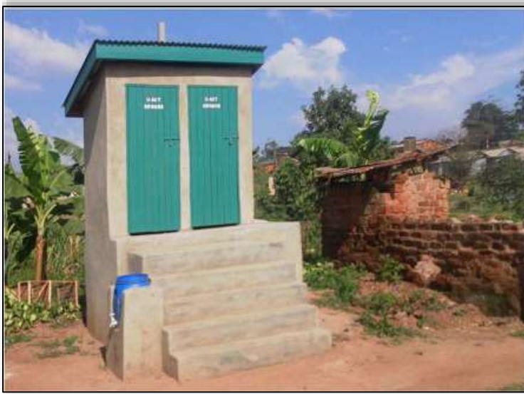
Figure 25-7 Front view of raised pit latrine
