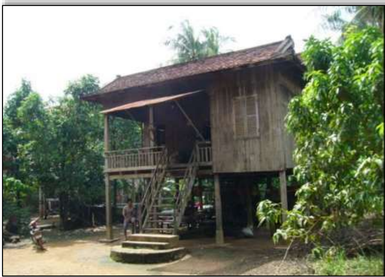
Figure 25-1 Wooden house on stilts
