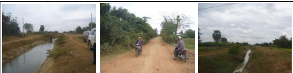
The existing canals, road, and social resources near the proposed landfill site-3
