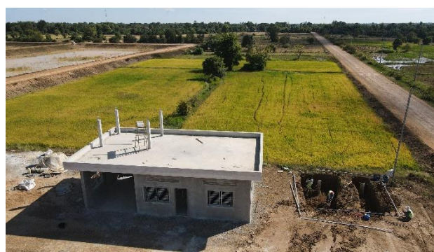
Overview of Workshop building at WWTP.
