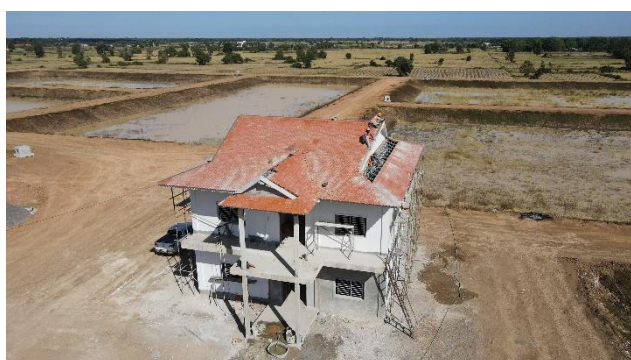
Overview of Administration building at WWTP.
