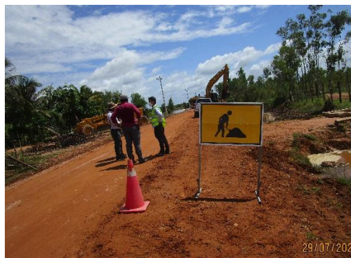
The clearing access road from NR No6 to landfill site. The access road will improve follow to existing road and will improve to concrete road
