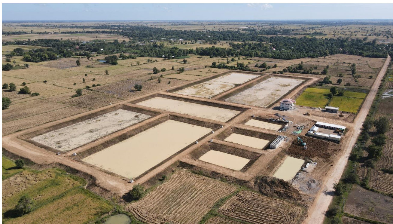
Overview of Wastewater Treatment Plant.
