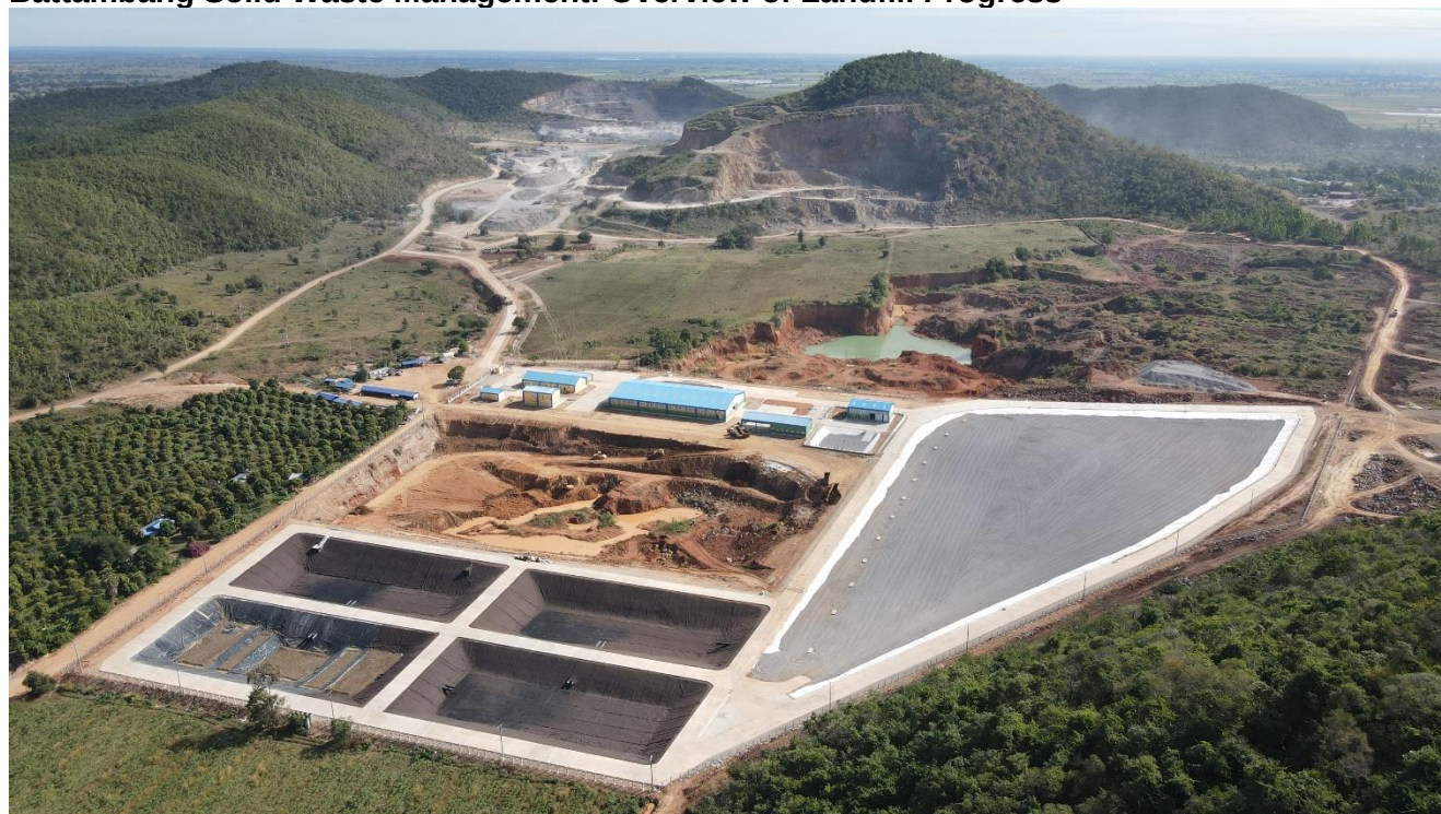
Battambang Solid Waste Management: Overview of Landfill Progress
