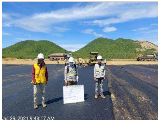
Asphal concrete pavement in cell 1 and finishing work of cell 1
