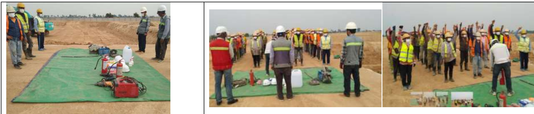
Training on Health and Safety and Emergency Procedures
