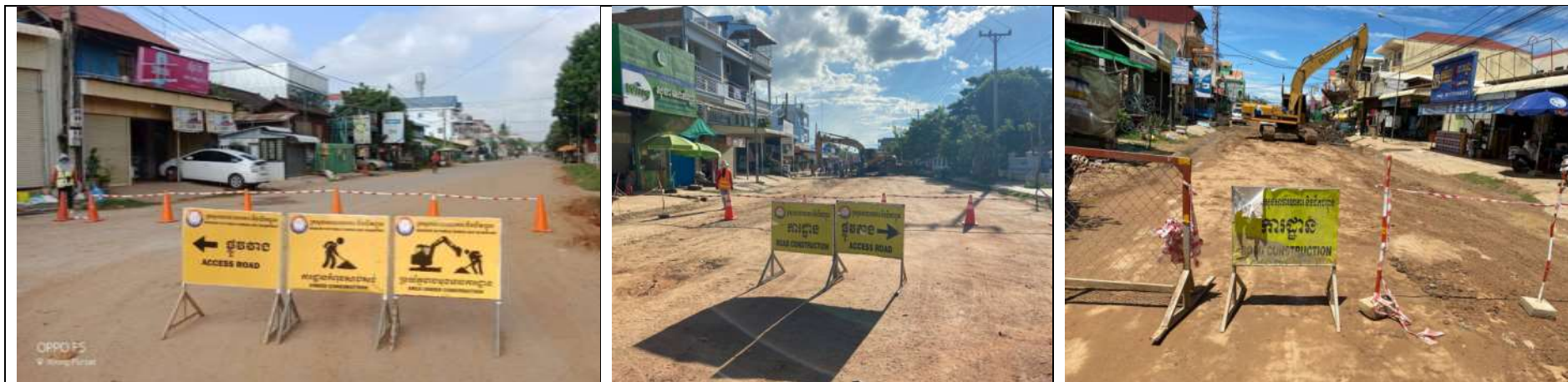
Traffic signs in construction site
