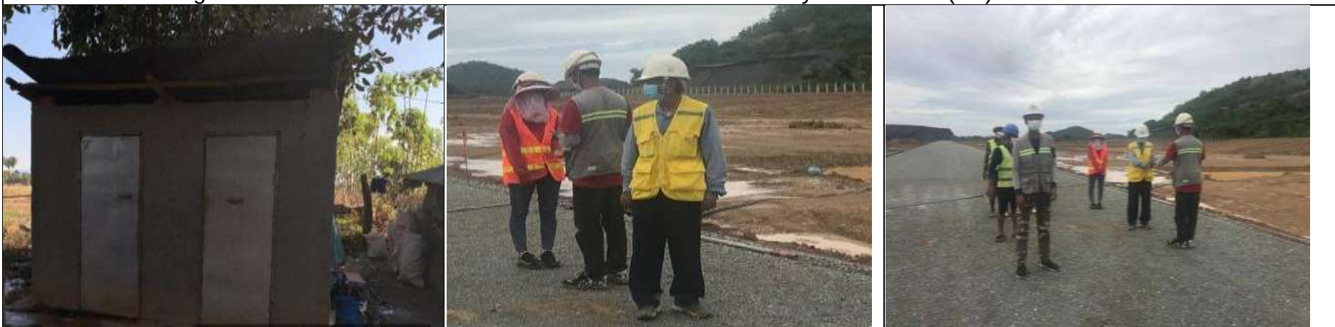
New toilets (Corrective Action Plan)
