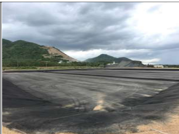
Asphal concrete pavement in cell 1 and finishing work of cell 1
