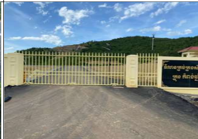
Finishing of main gate of landfill
