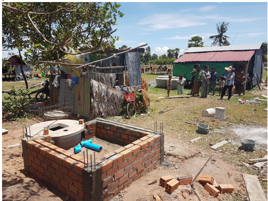
Photo 4-10: VIP latrine under construction in Toul Mkak village
