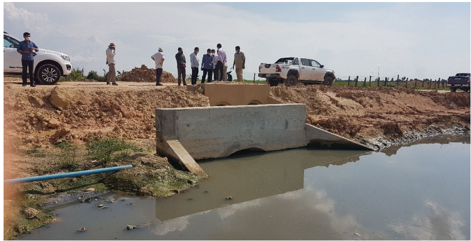
Photo 4-4 High level of backwater in front of the drainage outfall in the irrigation canal
