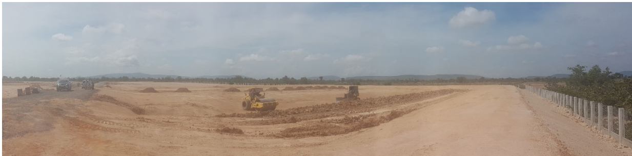
Photo 4-7: Overview of the Pursat Landfill Construction
