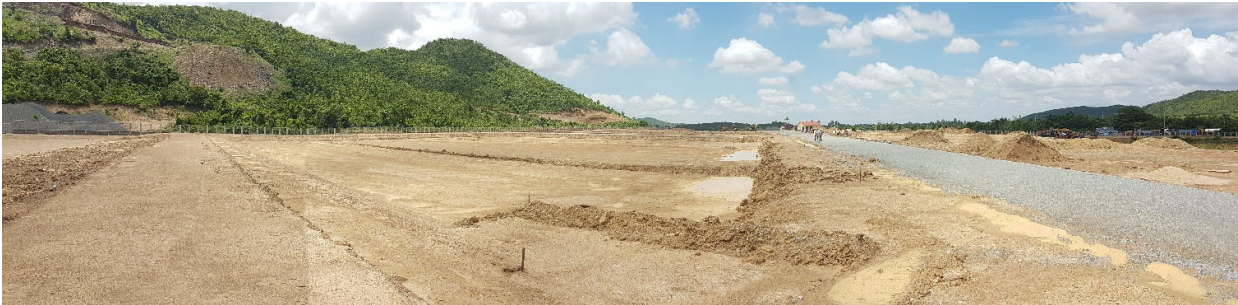
Photo 4-1 Overview of the landfill cell under construction
