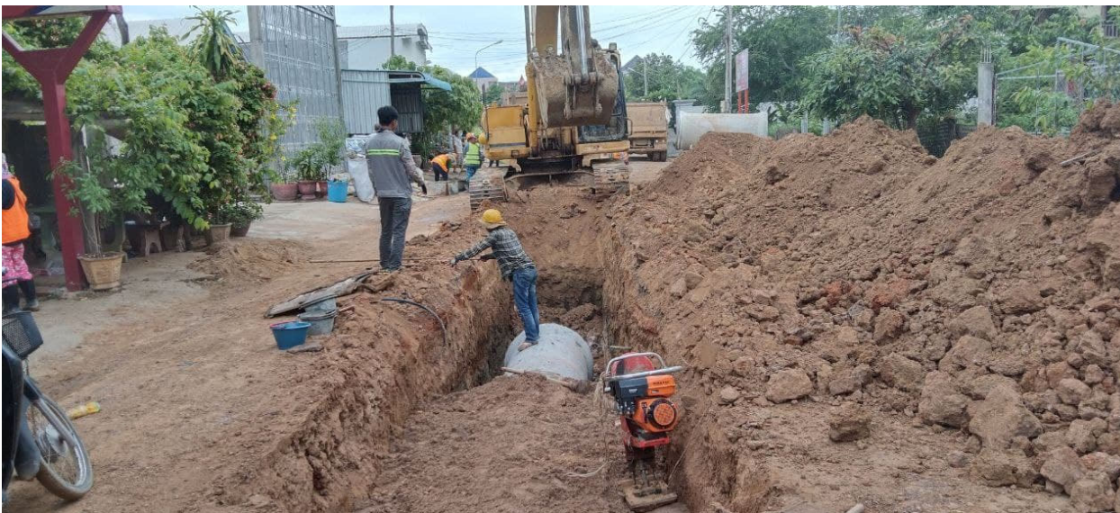
Photo 4-2: Installation of new drainage pipelines in the town center
