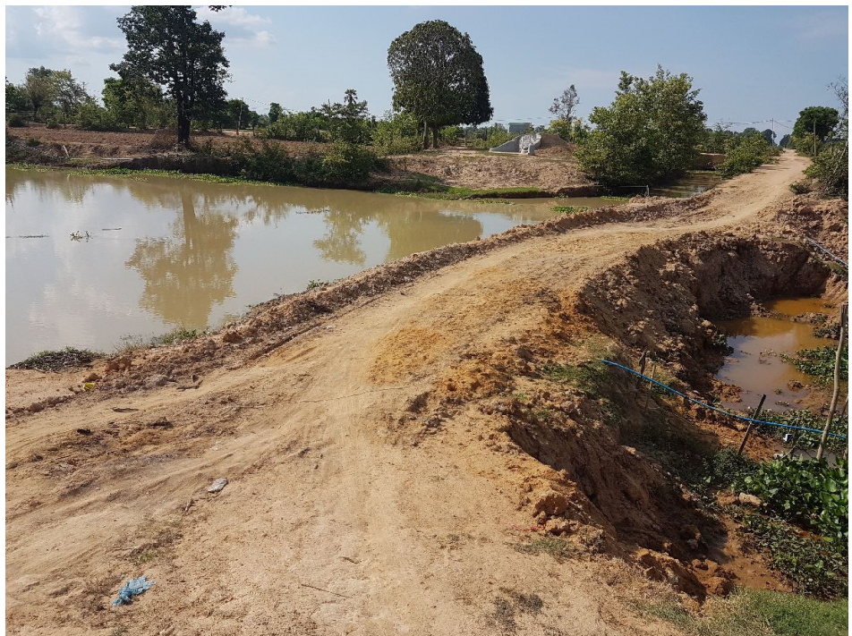
Photo 4-6 Dam in natural drain constructed by the local commune to protect the drain as source of drinking water
