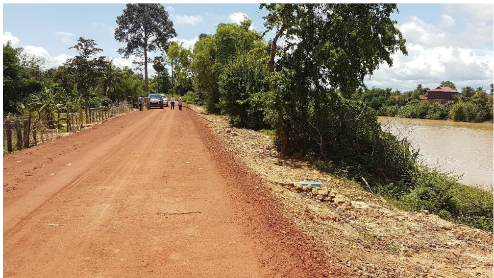
Photo 4-9: Reconstructed section of the river embankment
