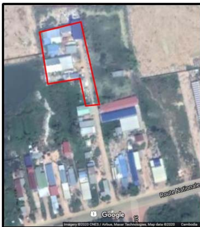
Figure 8: Aerial view of the first commercial MRF visited in Bavet. (coordinates 11° 3'0.21"N, 106° 4'42.21"E)
