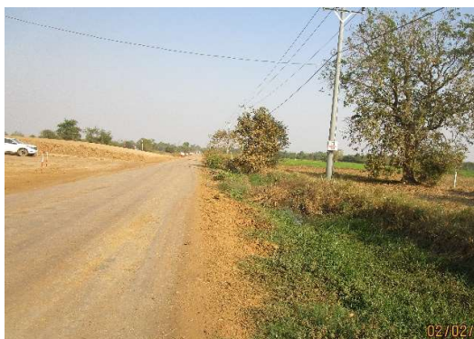
03-Feb-2021 Existing access road to WWTP site, BTB subproject
