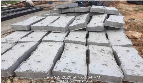
View of activities Pre-Cast of U-Drain making at the Yard in June 2020
