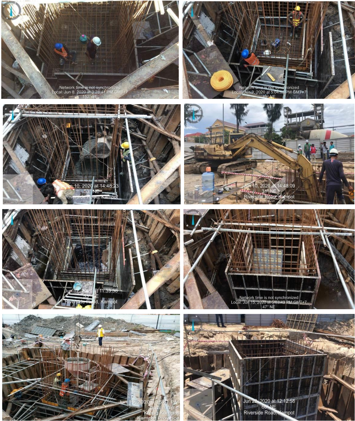
View of activities at the Pumping Station (C1) in June 2020
