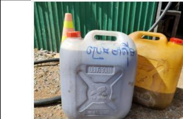
d. used oil for reuse to lubricate forms for precast slab and U-drain
