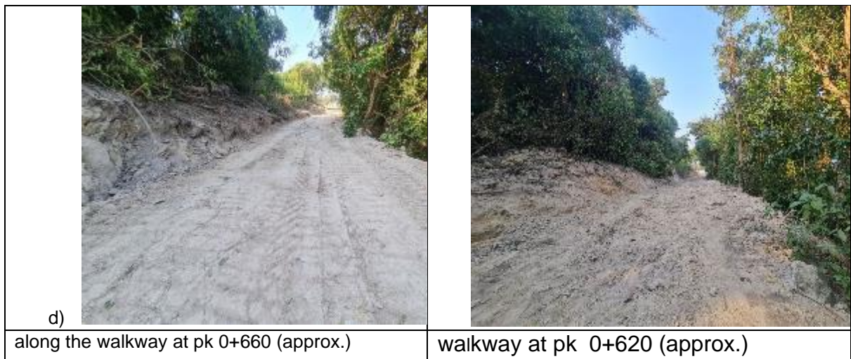
Figure 8. Initial land clearing and earthworks in Koh Tonsay Passenger Pier – December 2021
