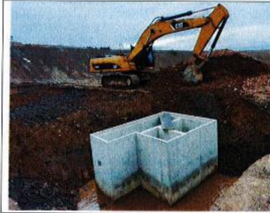
d. Construction of r.c. structures for Control Flow rooms and Excavation work for the wetlands
