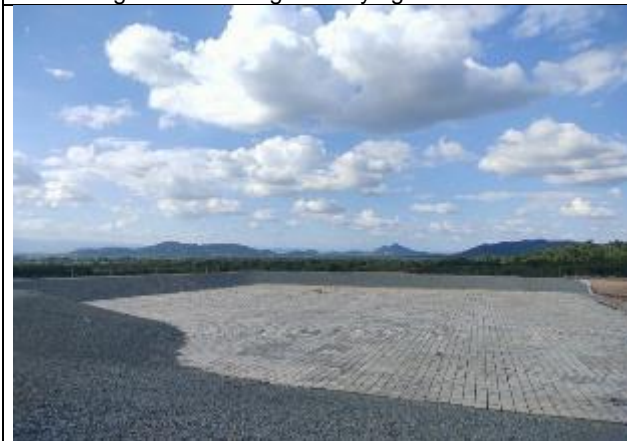
c. Protection of Cell bottom with concrete slab
