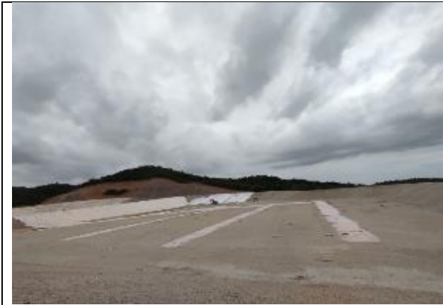
a. geotextile and gravel laying in Cell 4
