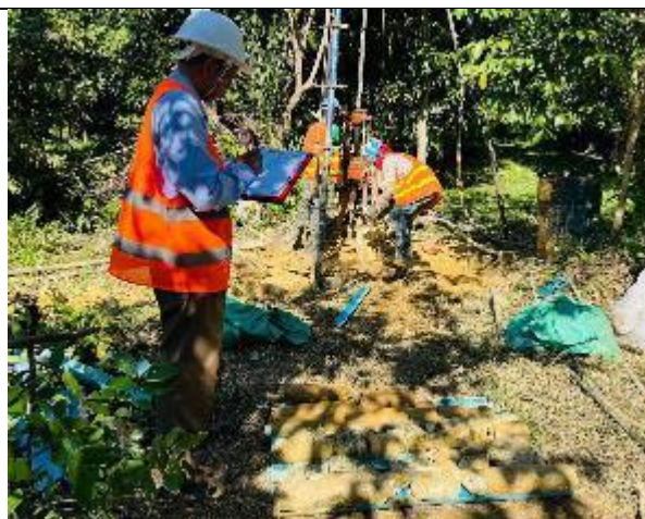
Drilling of well no. 2
