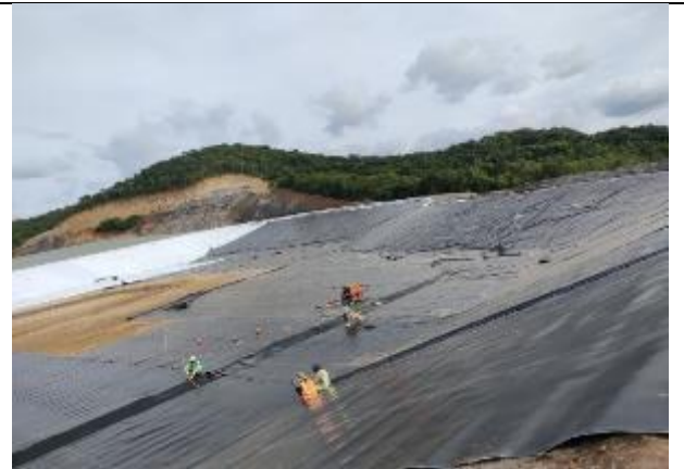
b. installation of HDPE in Cell 4
