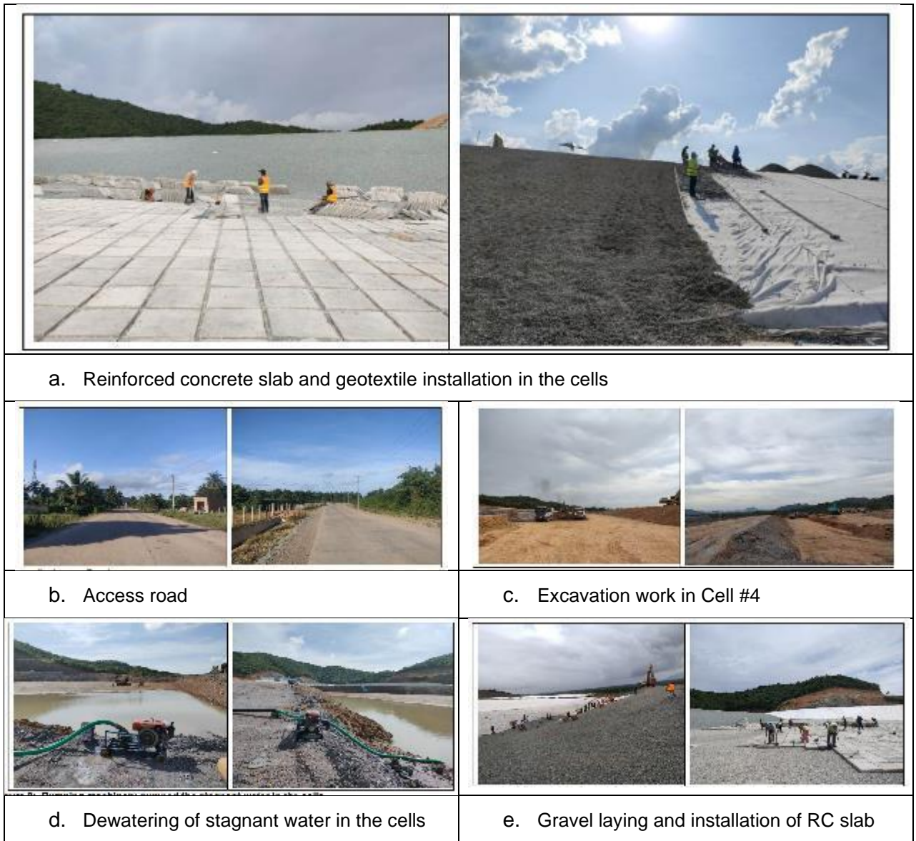
Figure 4. Kep CLF Project Site, October 2021
