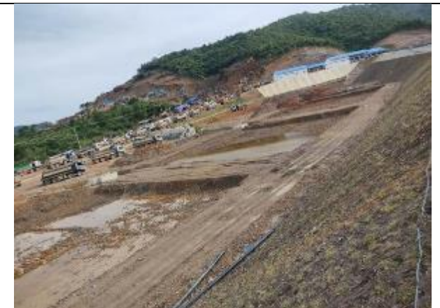
d. excavation works at the treatment and wetland areas
