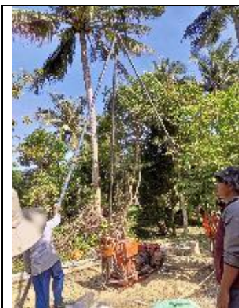
Drilling of well no.01
