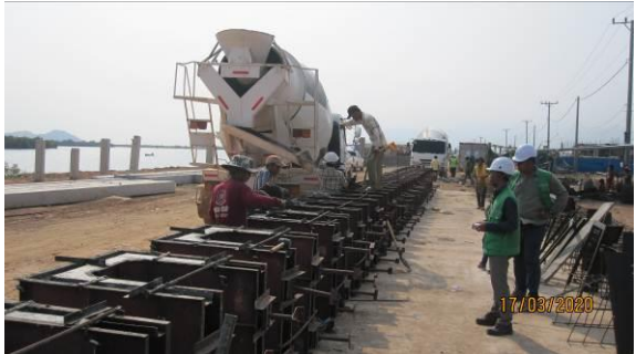
View of site visit the progress of construction works and supervising pre-cast construction of U-Drain in KPT on 19 Feb. 2020
