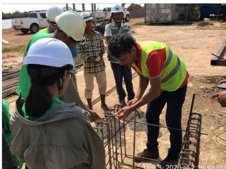
Frame bar of cover and U-Drain pre-cast making in the yard
