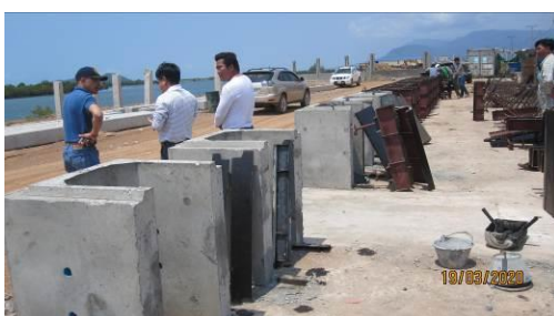
View of U-Drain mold and concrete works at the yard of the Contractor
