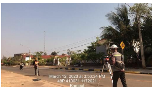
View of activity re-leveling works for all Lines of U-Drain
