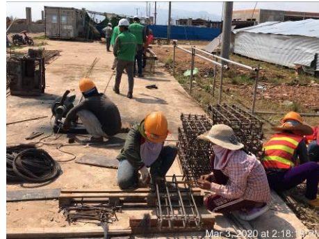
Frame bar of cover and U-Drain pre-cast making in the yard
