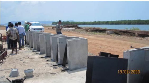
View of Pre-cast U-Drain construction at the yard of the Contractor
