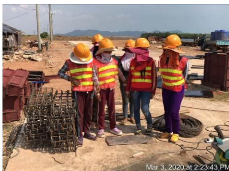
Frame bar of cover and U-Drain pre-cast making in the yard
