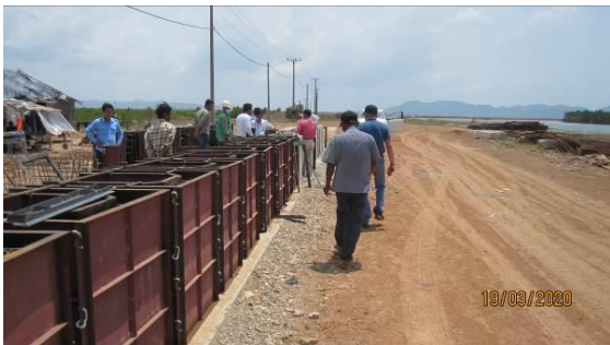
View of Pre-cast U-Drain construction at the yard of the Contractor
