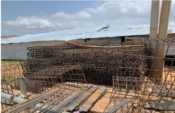
View of frame bar and molds preparation for Pre-cast concrete work
