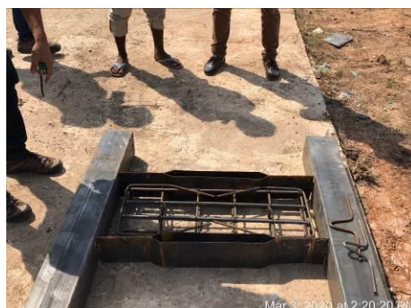
Frame bar of cover and U-Drain pre-cast making in the yard
