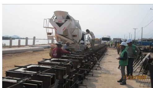
View of U-Drain mold and concrete works at the yard of the Contractor
