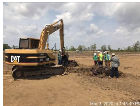
Soil excavation test of the bottom of WWTP site
