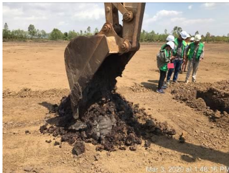
Soil excavation test of the bottom of WWTP site
