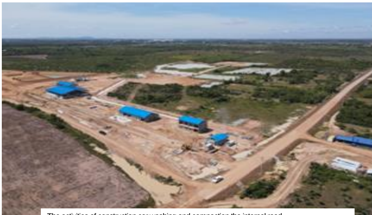
The activities of construction car washing and compaction the internal road
