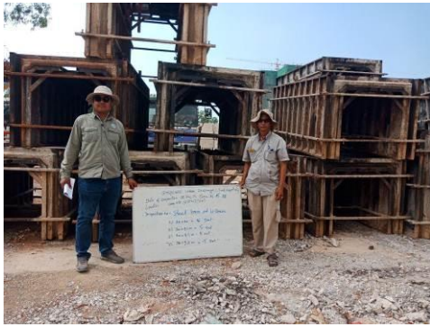
007..The quantity Steel form of U-Drain The quantity Steel form of covers
