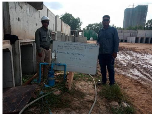
008... Well Drilling and Pump
