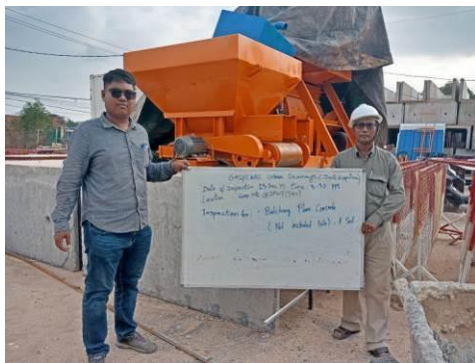
005.. The Concrete Batching Plant
