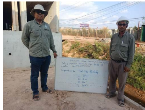
015.. Slab for pre-cast concrete
