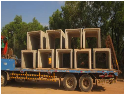
View of U-Drain mobilization from the public site to the Yard of WWTP, SHV Photos of Activities Site preparation for Camp at MPS, CW01 sub-project in KPT
