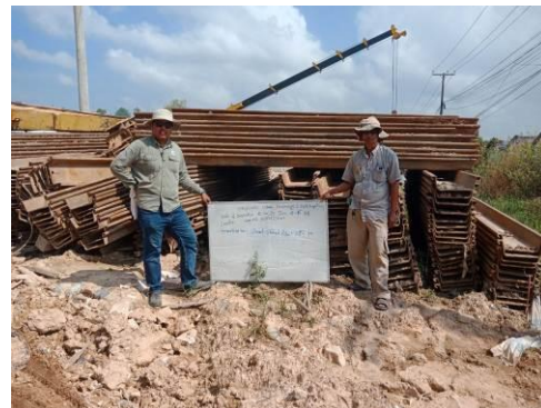
012..The quantity of Steel sheet piles
