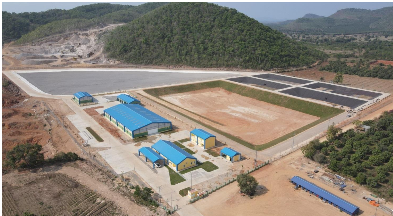
View from drone on the Landfill site
