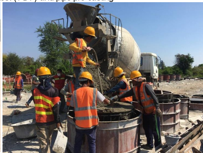
The activities of the sub grade soil test ( FDT ) and pipe pre-casting
