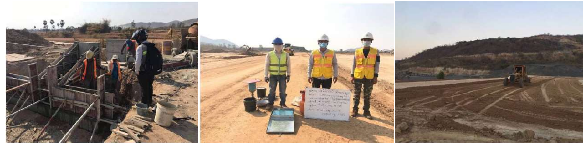
Construction activities at landfill site
