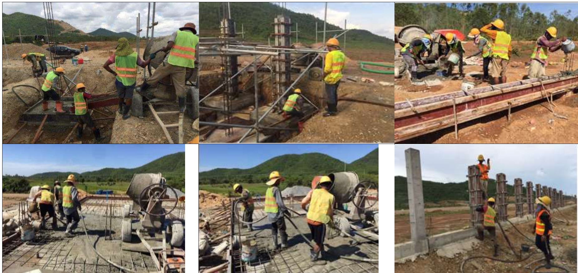
Construction work equip with PPE during working in construction site
