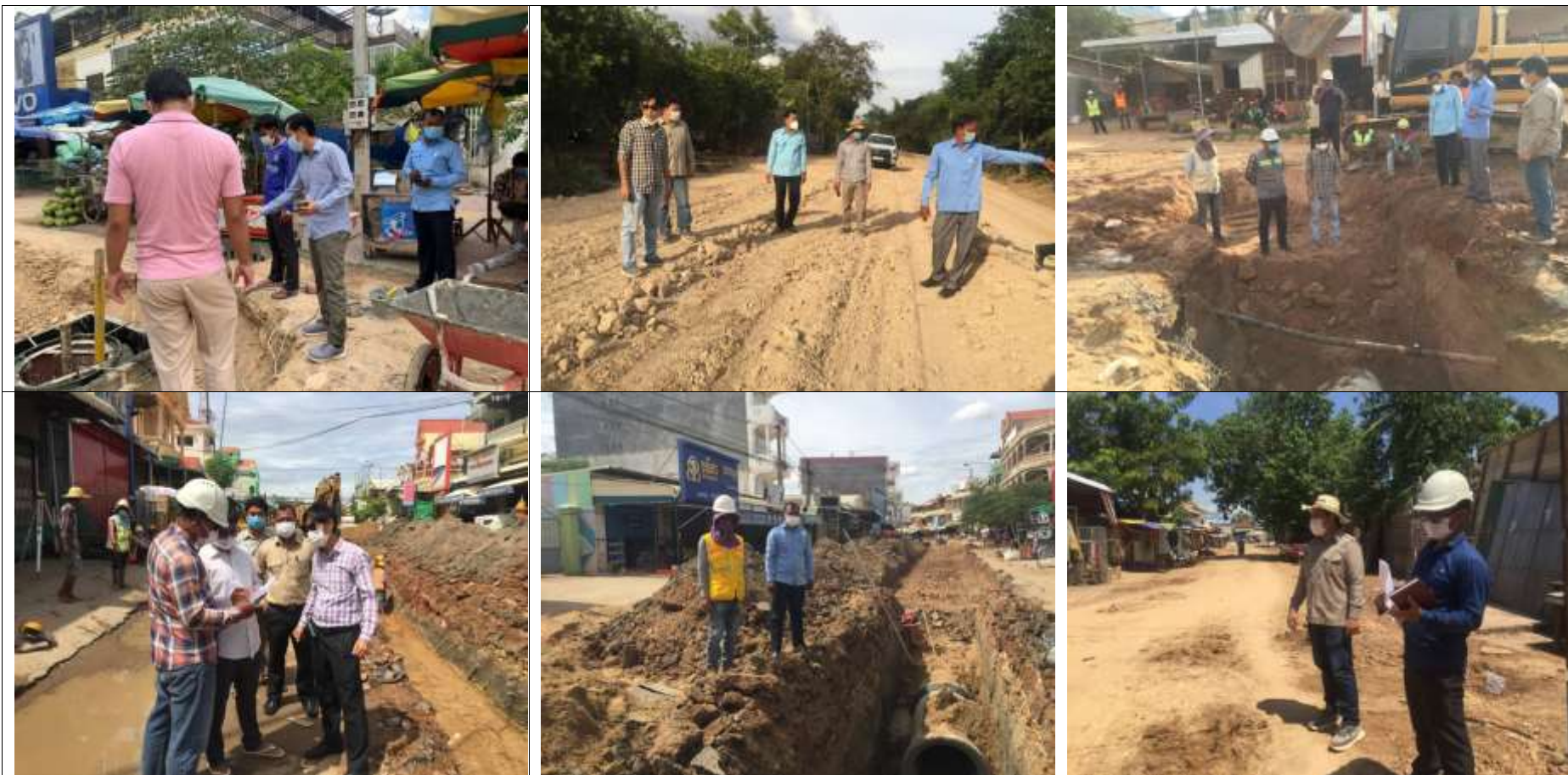
Site observation from PIU team during construction period at drainage site
