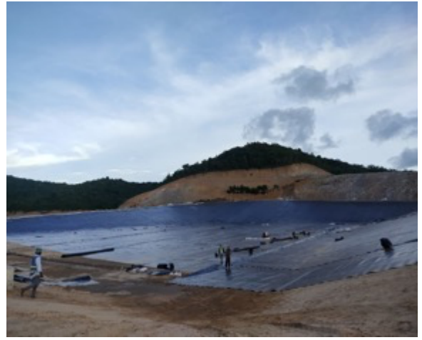
Installation Geotextile in Cell 3
