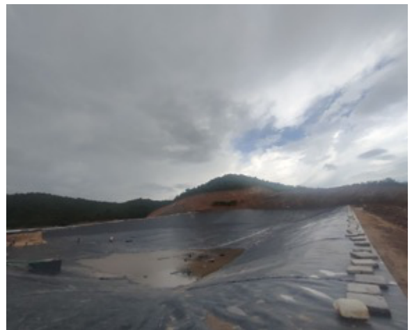
Installation of HDPE Liner in Cell 3
