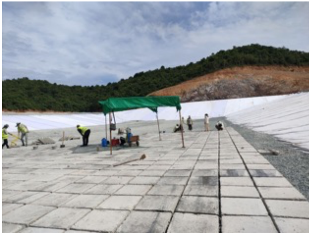
Installation Precast R.C Slab in Bottom of Cell 2
