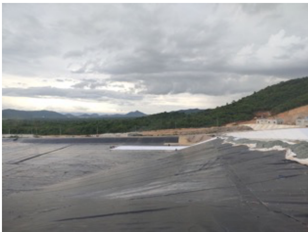
Installation of HDPE Liner in Cell 3
