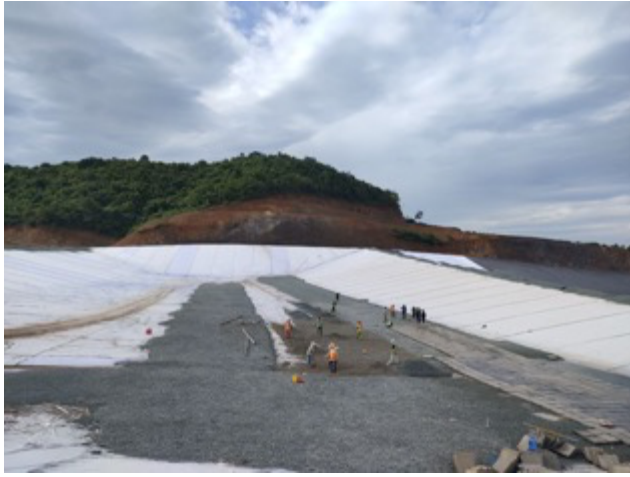
Installation Precast R.C Slab in Bottom of Cell 2
