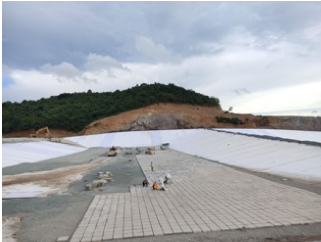
Installation of HDPE Liner in Cell 3
