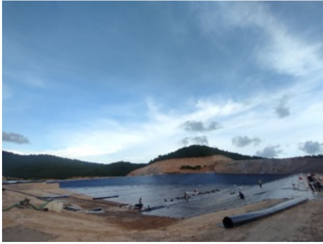
Installation Geotextile in Cell 3
