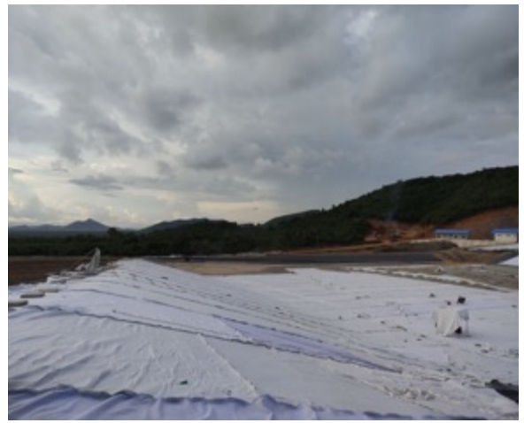
Installation Geotextile in Cell 3
