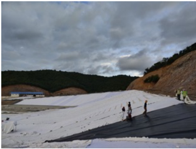
Installation Geotextile in Cell 3
