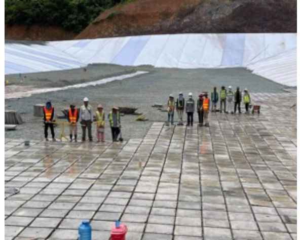
Installation of HDPE Liner in Cell 3
