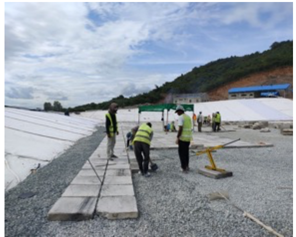
Installation Precast R.C Slab in Bottom of Cell 2
