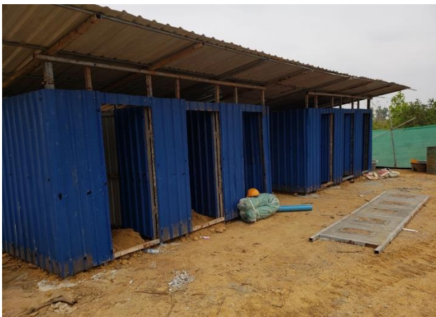
Camp Site, Equipment for Kratie landfill project: PMC and Contractor KBH
