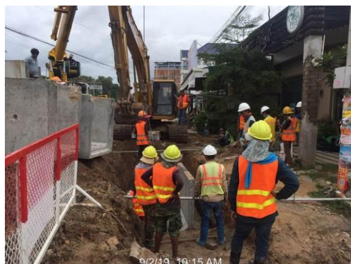
The clearance, excavation, and installation U-D activities on line 15 (road #810)
