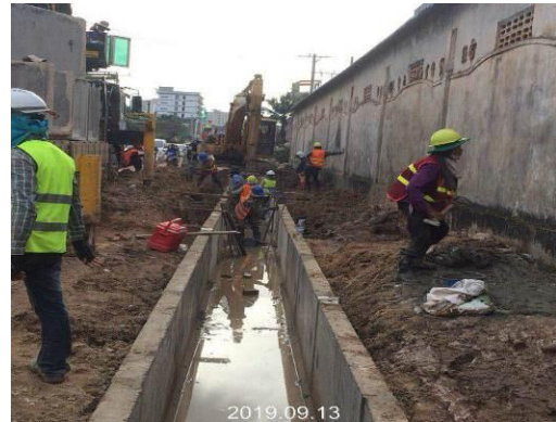
The clearance, excavation, and installation U-D activities on line 14 (road #104)
