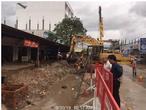
The clearance, excavation, and installation U-D activities on line 19 (road #8144)
