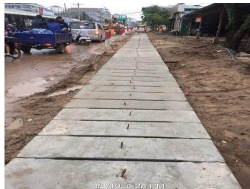
The clearance, excavation, and installation U-D activities on line 19 (road #8144)
