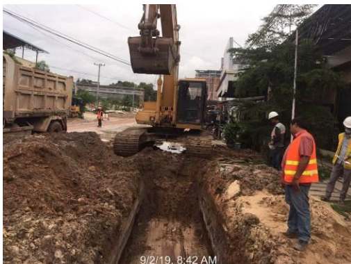
The clearance, excavation, and installation U-D activities on line 19 (road #8144)
