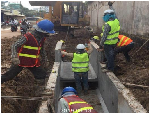
The clearance, excavation, and installation U-D activities on line 14 (road #104)
