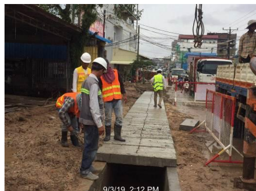
The clearance, excavation, and installation U-D activities on line 15 (road #810)
