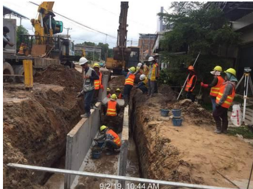
The clearance, excavation, and installation U-D activities on line 19 (road #8144)
