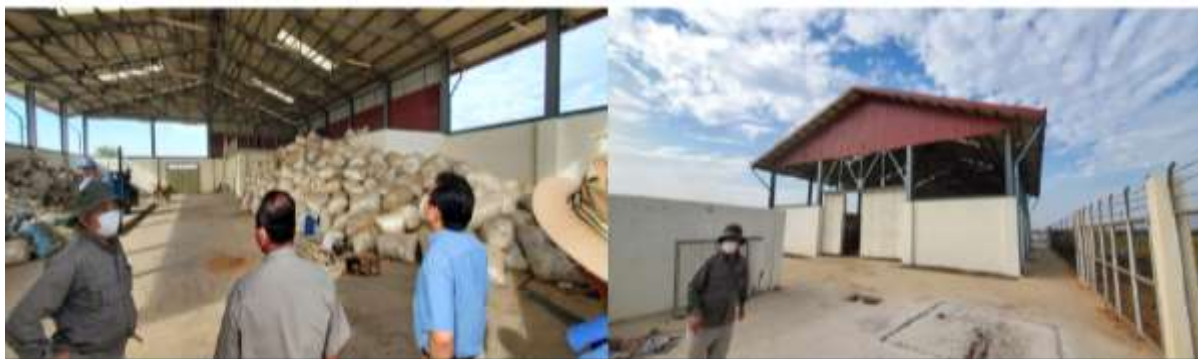
Figure 5: The Materials Recovery Facility at the Existing Dumpsite
