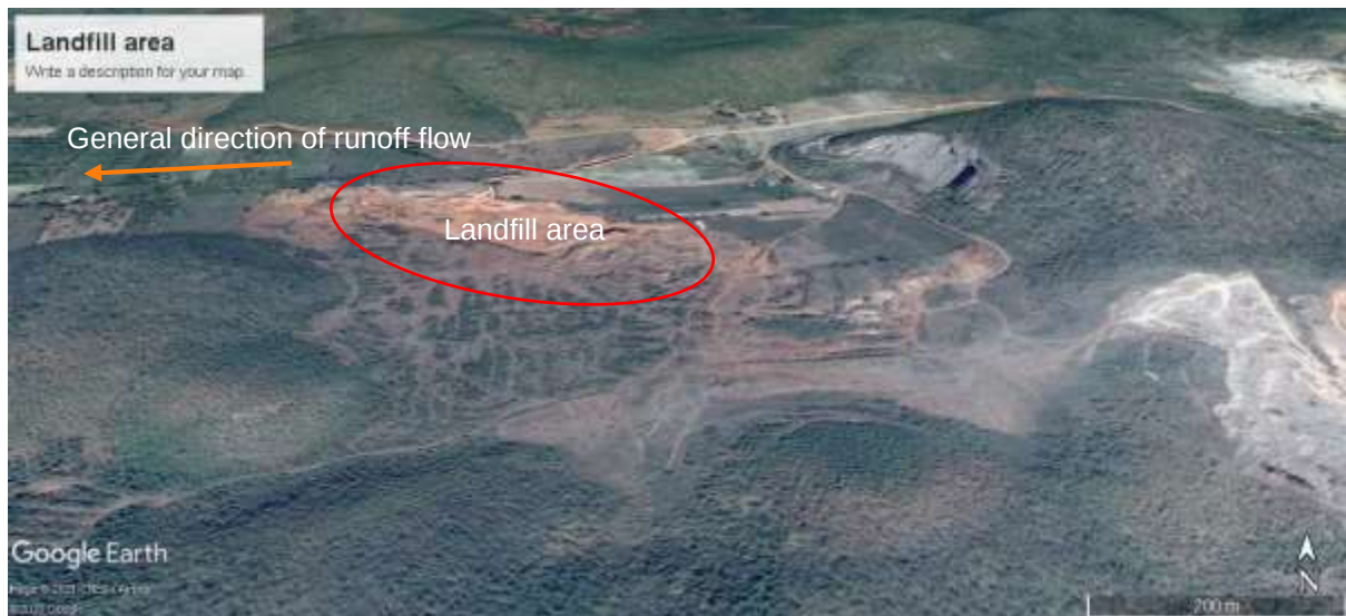
Figure 28: Google Earth Image (April 2017) of the Landfill Area
