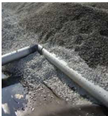
Figure 18: Leachate Collection System within the Cell
