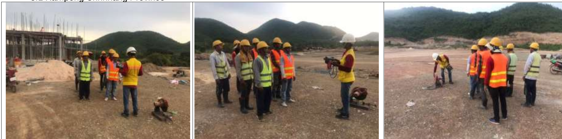
Training to unskill workers on how to use cutting equipment
