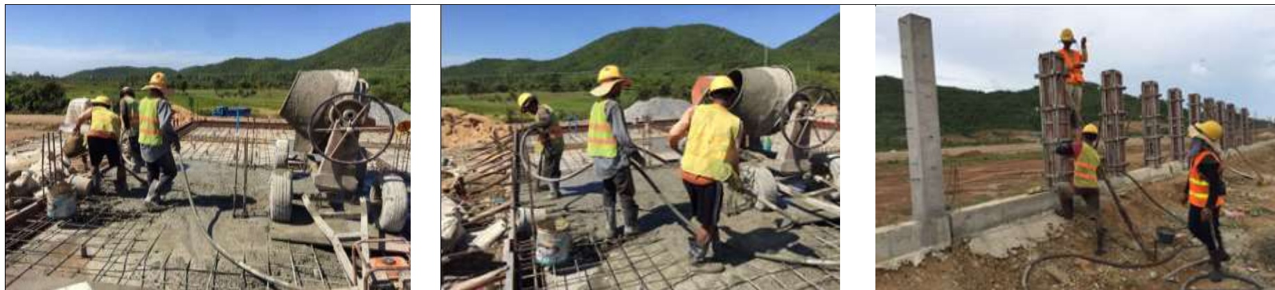
Construction work equip with PPE during working in construction site
