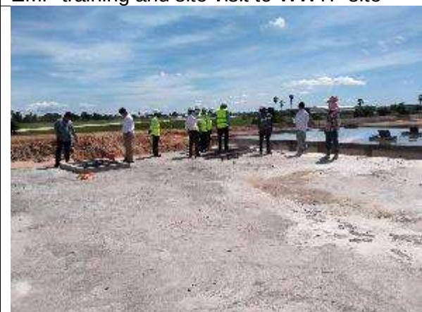
EMP training and site visit to WWTP site
