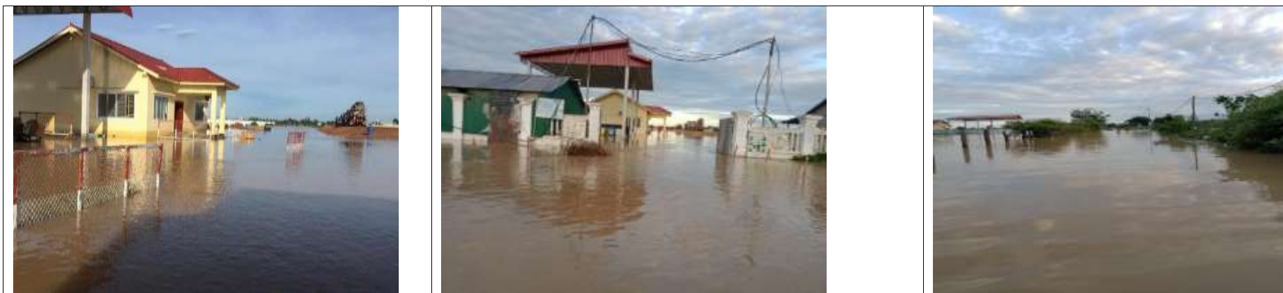
High flood during September and October 2020 at WWTP Pursat province
