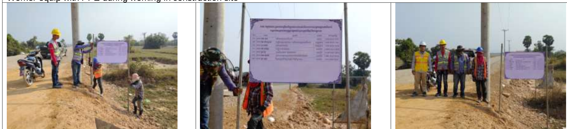
GRM sign board installation at construction site
