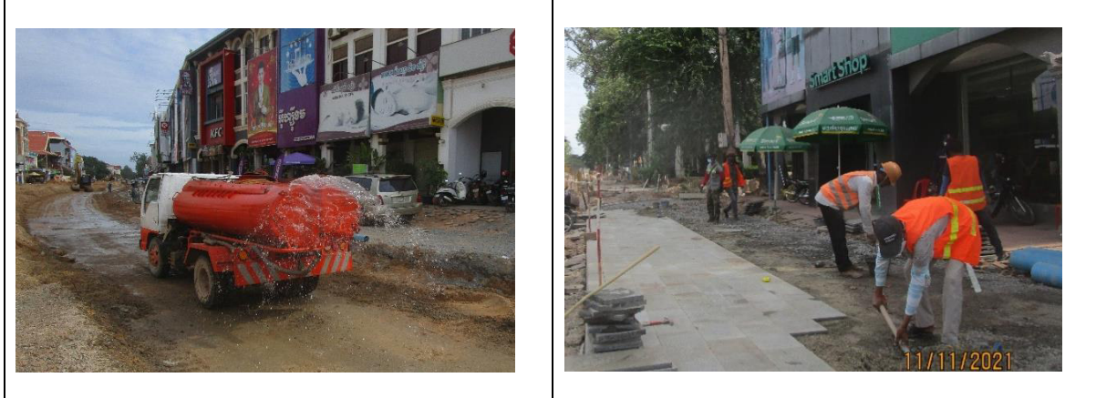
The present of road construction activities in November 2021
