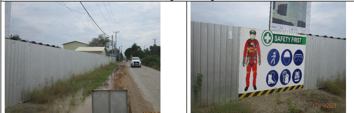
Fencing construction campsite with safety sign boards
