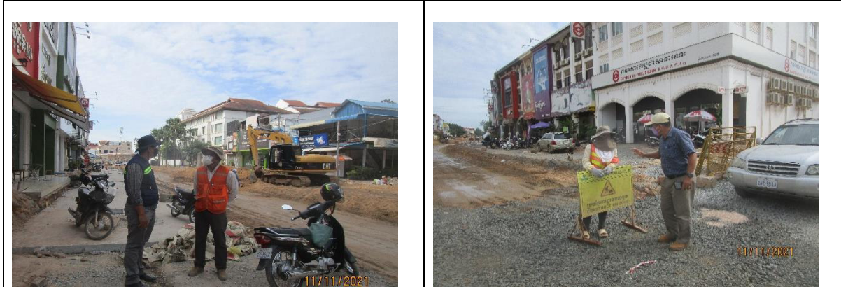
Discussed with site engineer and construction worker
