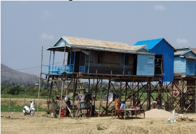
Houses erected in new location in Chong Kosh-02
