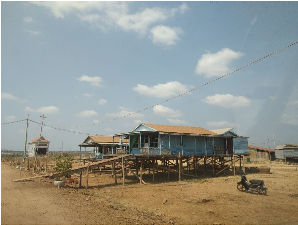
Homes erected in new location in Chong Kosh-01
